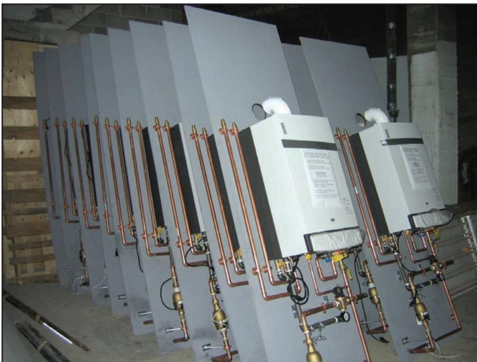
*To ensure quality and reduce installation time, Westcorp first mounts each Baxi unit on a 6-foot-high board in a heated warehouse on the construction site. Boilers are piped for easy connection to gas and water supplies, and the hydronic systems.*
